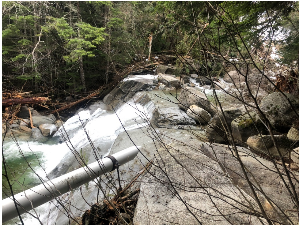
Photo looking at prior intake location. Note that intake is downstream of debris lobes suggesting that release flooding likely washed away in-stream structures.
